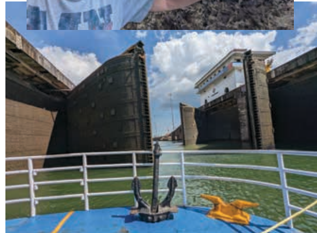
right: The last lock before the Pacific Ocean. This is the original lock from the construction in 1914
