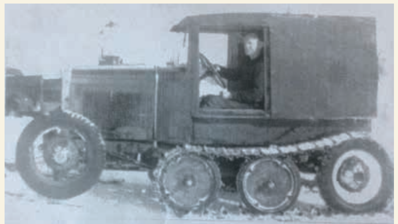
George Thompson, relief mail carrier, created a truck "snowmobile" with skis in front and tracks in the back.
